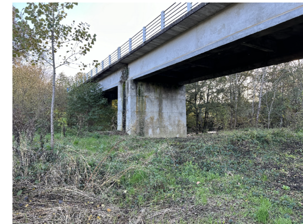
DESERBAGE, NETTOYAGE OA EXISTANT TRAITEMENT JOINT EXISTANT
