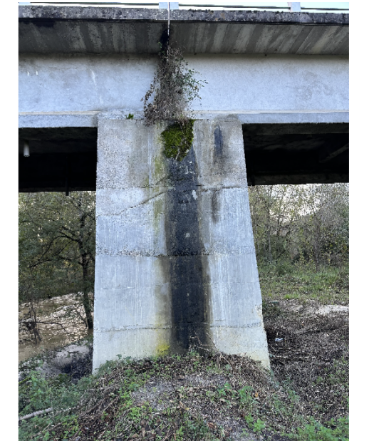
DESERBAGE, NETTOYAGE OA EXISTANT TRAITEMENT JOINT EXISTANT
