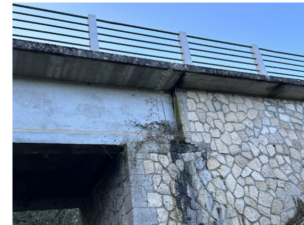
DESERBAGE, NETTOYAGE OA EXISTANT TRAITEMENT JOINT EXISTANT
